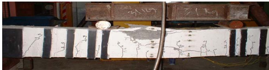
Plate 3. Failure mode of beam C4 (CFRP laminate strengthened beam with L shape end and intermediate anchorages)
