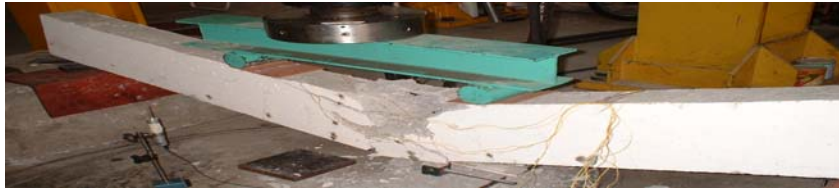
Plate 1. Failure mode of beam A1 (Control beam)
