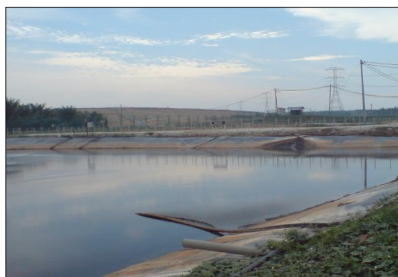
Figure 4: Leachate treatment plant in Jeram landfill
